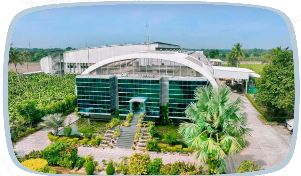
Motor manufacturing facility, India
