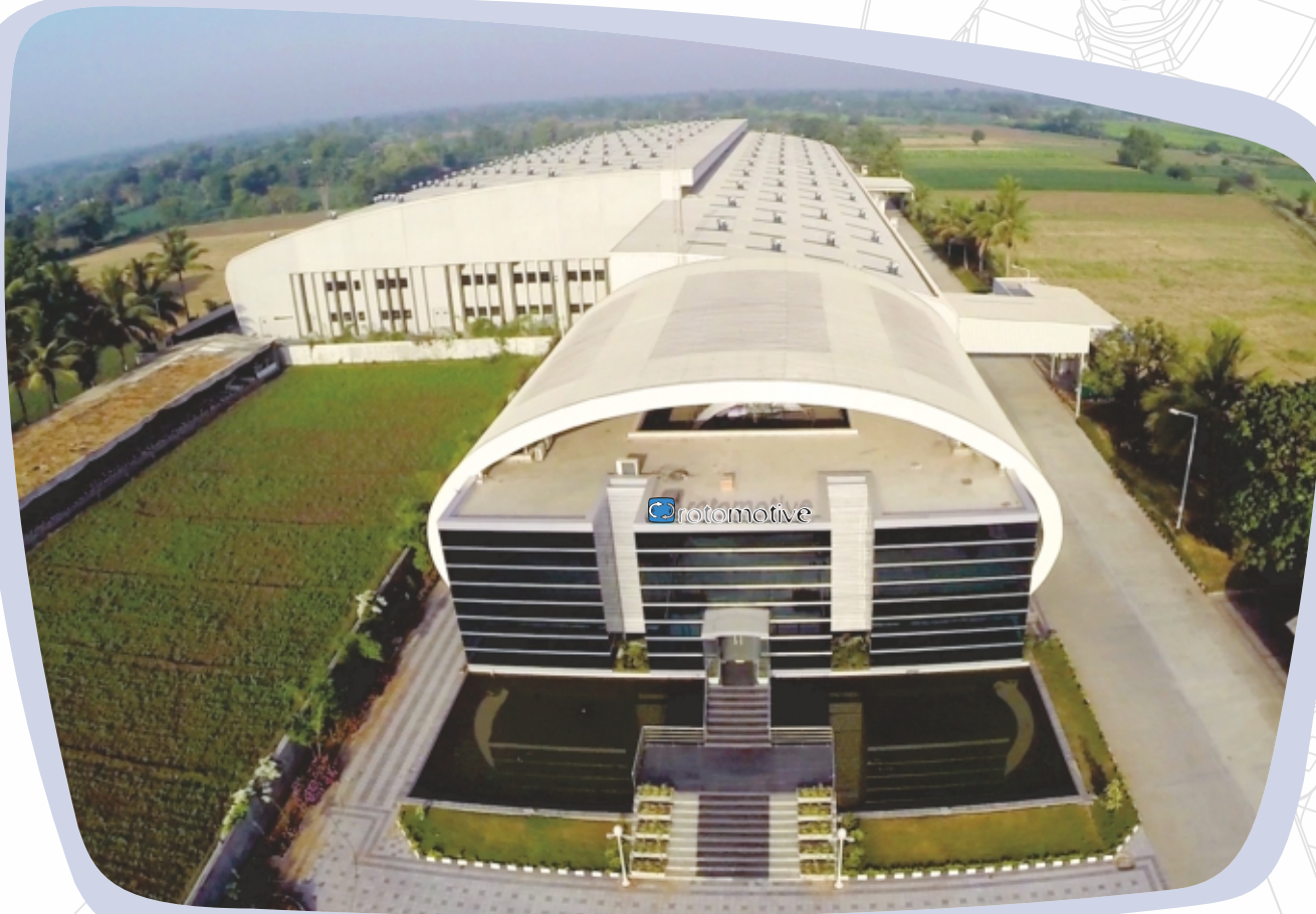
Our Manufacturing facility in India
